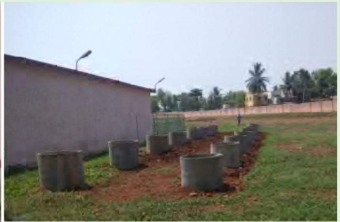
Installed Cemented Rings
