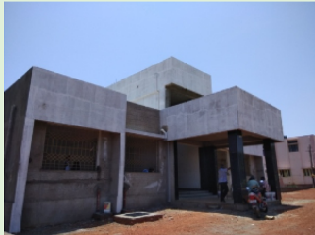
Laboratory cum office building works in progress
